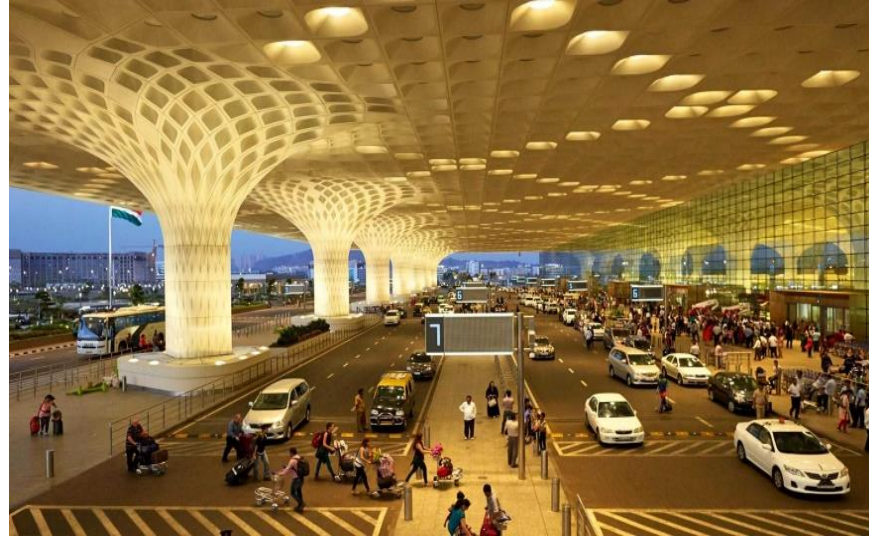
MUMBAI INTL AIRPORT – T2 TERMINAL (2012)
