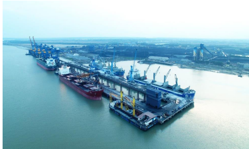
DHAMRA PORT, ODISHA (2019)
